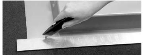
3) Since the Drip Tray fits over the face frame and in most cases a center mullion, you will need to trim Drip Tray to fit flush to the front. A utility knife may be used to make the cuts, but a power tool (jig saw, scroll saw, etc) might give you a little more control.
