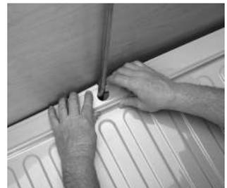
5) Use silicon adhesive around the entire perimeter and any holes you made for plumbing. Take care to seal all the cuts to ensure a water tight seal.
