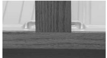
4) Once tray is fitted inside cabinet, use silicon adhesive around the entire perimeter and any holes made for plumbing. Take care to seal all the cuts to ensure a water tight seal.
