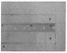
Screw the aluminum bracket into the studs and reinforcement beam. Make sure the groove is facing up and is level.
