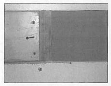
3. Install a 2 x 8 beam between two (or more) studs, depending on the width of the vanity.
