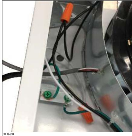
❸ Strip the end of the 3 wires from GREY cable (the one with ferrite), then using small UL approved wire nuts (suitable for 22 AWG wires), connect these wires with ADA cable wires. Connect as follows: WHITE wire with WHITE wire, BLACK wire with BLACK wire and RED wire with RED wire.
